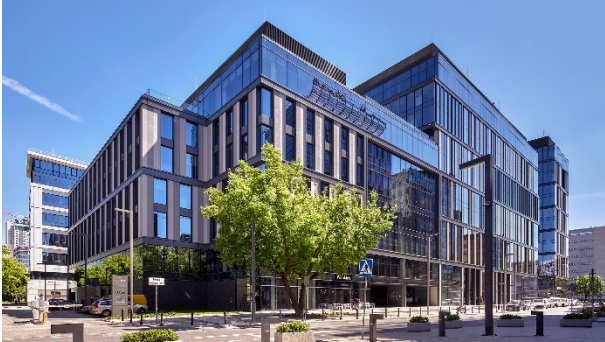
Proximo II administrative building, Warsaw, Poland
