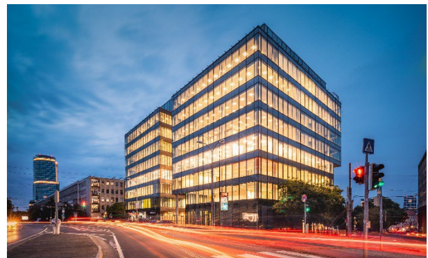
Administrative building Park One, Bratislava, Slovakia
