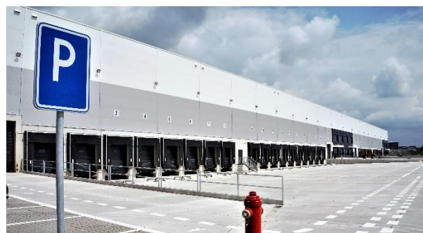
Industrial Park Sered' DC32, Sered', SR
