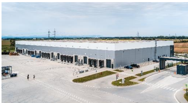
Industrial Park Sered' DC31, Sered', SR
