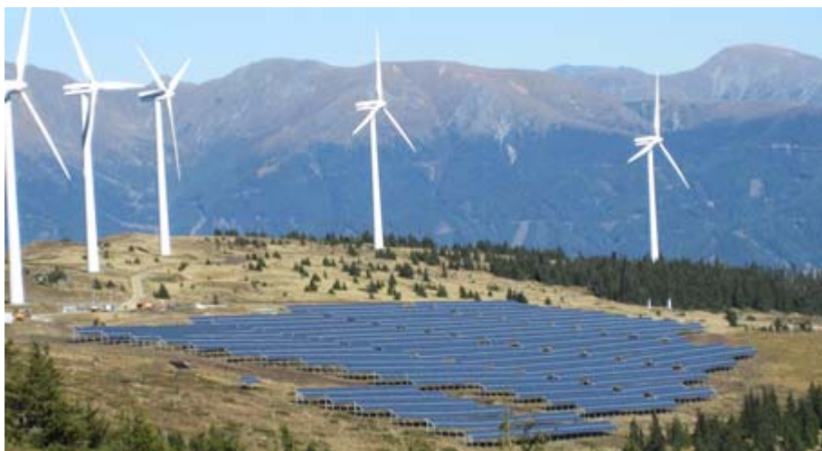
photovoltaic power plant at Lower Tauern (Styria)
